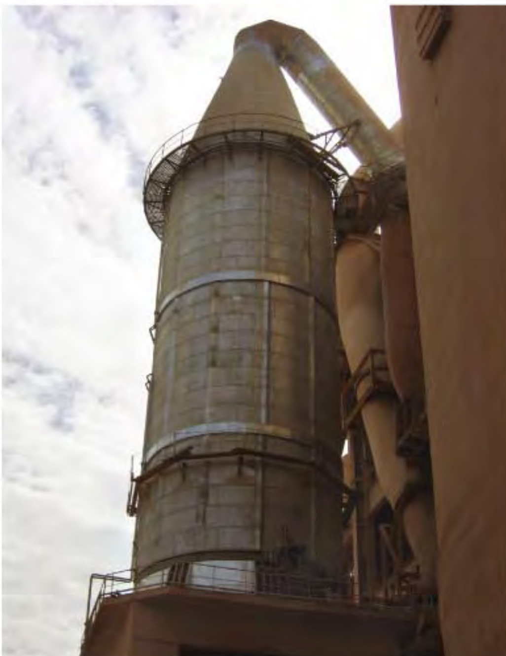
A Gas Conditioning Tower install in a cement plant at Belgium.
