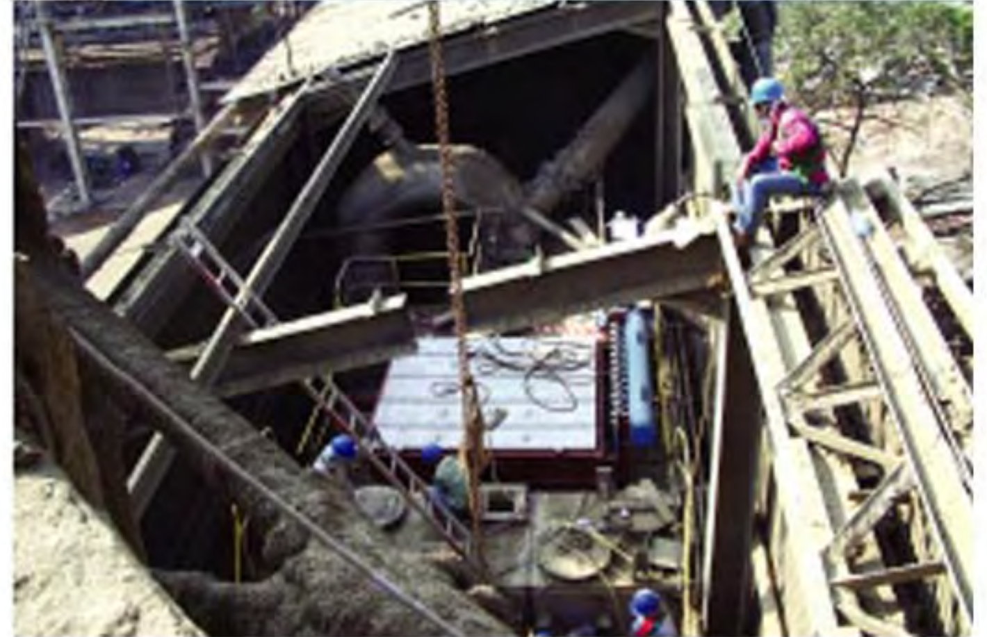
A Conversion of Electrostatic Precipitator to Fabri-Pulse Filter Job done for Lafarge, Malaysia.
