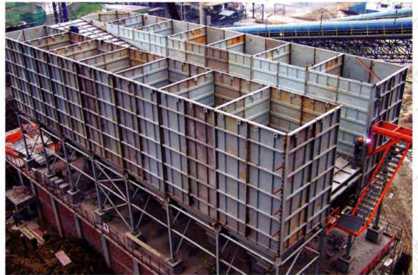
AAF Fabri-Pulse XLC bagfilter during site erection stage.
